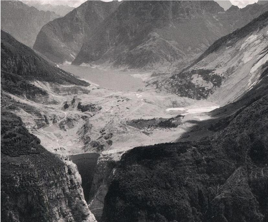
Figure 8.2 | An image of the Vajont reservoir shortly after the massive landslide (landslide scar at right, dam located in foreground on the left). Source: Unknown (1963) copyright expired. view source
