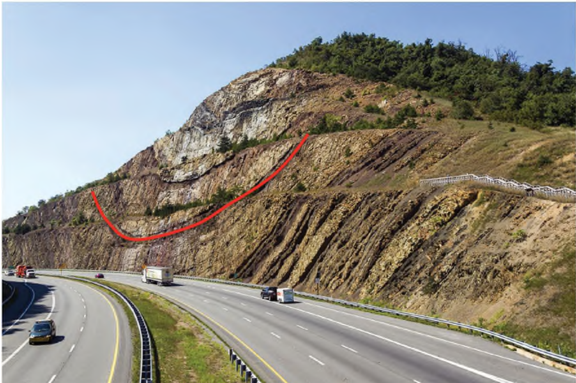
Figure 8.19 | This road cut shows a cross-section through a syncline ("U" shaped fold). It is located along Interstate 68 and US 40 in Maryland, USA. Source: Wikimedia User "Acroterion" (2012) CC BY-SA 3.0. View Source .
