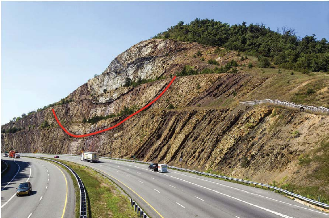
Figure 8.19 | This road cut shows a cross-section through a syncline ("U" shaped fold). It is located along Interstate 68 and US 40 in Maryland, USA. Source: Wikimedia User "Acroterion" (2012) CC BY-SA 3.0. View Source .
