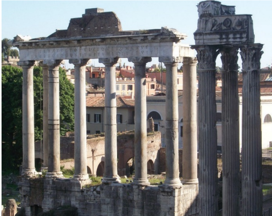
Figure 8.15 | The Roman Forum. Why did the Romans use so many vertical columns to hold up the one horizontal beam? If the horizontal beam spanned a long distance without support, it would buckle under its own weight. This beam is experiencing tensional stress, and rocks have very little strength when exposed to such stress. Source: Randa Harris (2015) CC BY-SA 3.0 view source
