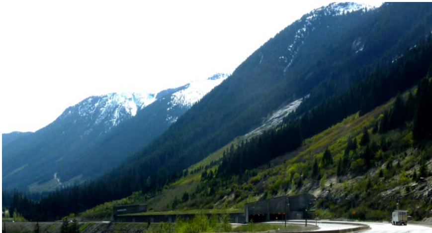
Figure 15.22 | A snow avalanche shelter on the Coquihalla Highway (bottom centre of the image). The expected path of the avalanche is the steep and treeless slope above.
