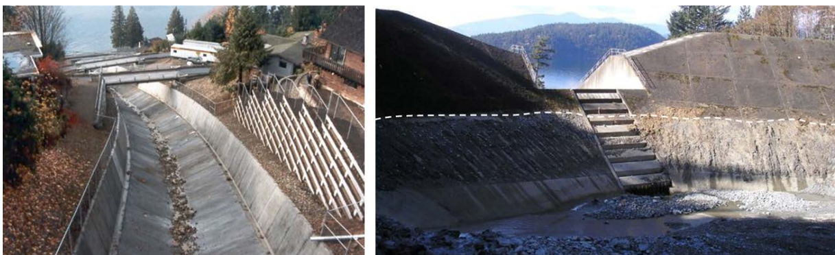
Figure 15.23 | Two strategies for mitigating debris flows on the Sea-to-Sky Highway. Left: A concrete –lined channel on Alberta Creek allows debris to flow quickly through to the ocean. Right: A debris flow catchment basin on Charles Creek. In 2010, a debris flow filled the basin to the level of the dotted white line. Source: Steven Earle (2015) CC BY 4.0. View source https://opentextbc.ca/geology/
