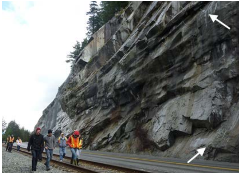
Figure 15.10 Site of the 2008 rock slide at Porteau Cove. Notice the prominent fracture set parallel to the surface of the slope. The slope has been stabilized with rock bolts (top arrow) and holes have been drilled into the rock to improve drainage (tube from drainage hole indicated with bottom arrow). Risk to passing vehicles from rock fall has been reduced by hanging mesh curtains (background), which secures loose material to the slope. Source: Joyce McBeth (2018) CC BY 4.0 after Steven Earle (2015) CC BY 4.0. View source https://opentextbc.ca/geology/
